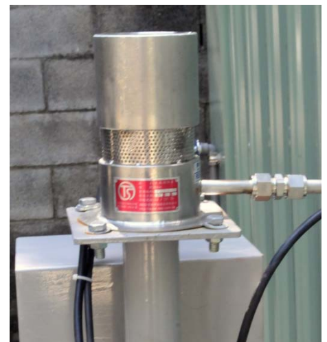
End of Line Flame Arrester, with Automatic Flare, was developed by RESI for Laboratory Applications.
